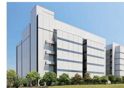
netXDC Chiba Center 3 (SI3)
